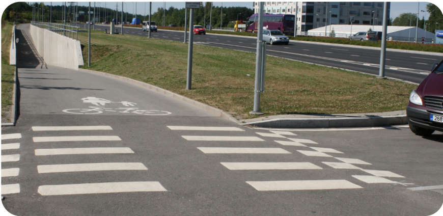
A cycle and pedestrian track with a threshold intersecting with a carriageway.
